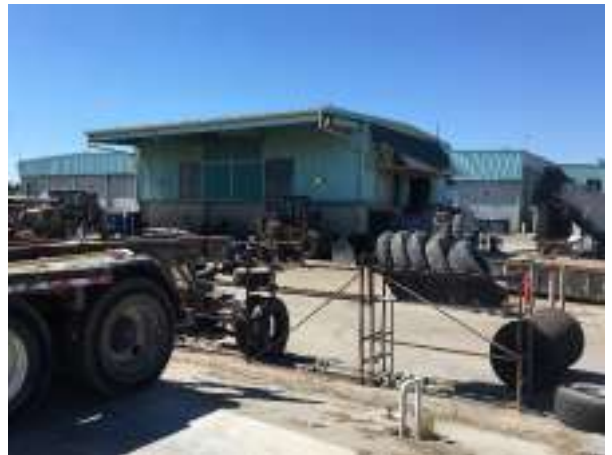
Figure 13. Maintenance Building with Storage
