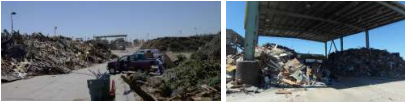
Figure 10. C&D and Green Waste Dropoff Area and C&D Tipping Building
