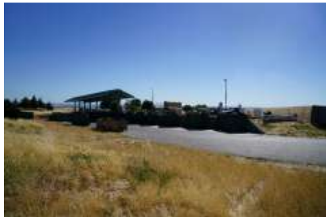
Figure 8. Z-wall, Public Tipping Area
