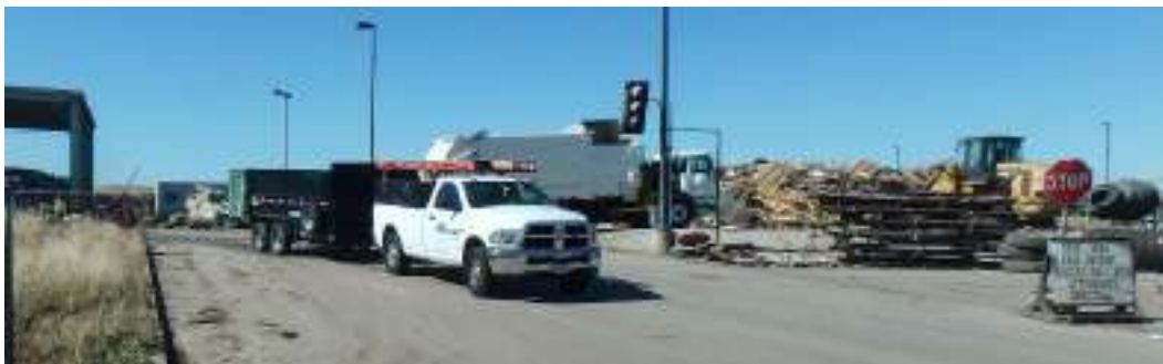
Figure 4. Proximity of Windrows to Incoming and Outgoing Traffic
